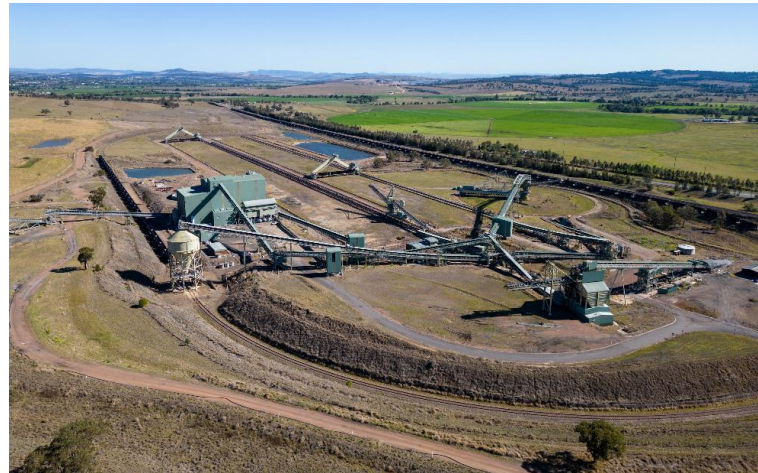
View of the Dartbrook mine surface infrastructure include the CHPP and rail siding
